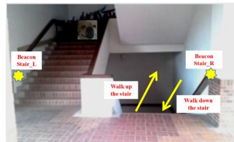
Fig. 3 Two beacons installed on the walls of a staircase.
